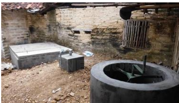
Figure 6. The finished biogas reactor unit
